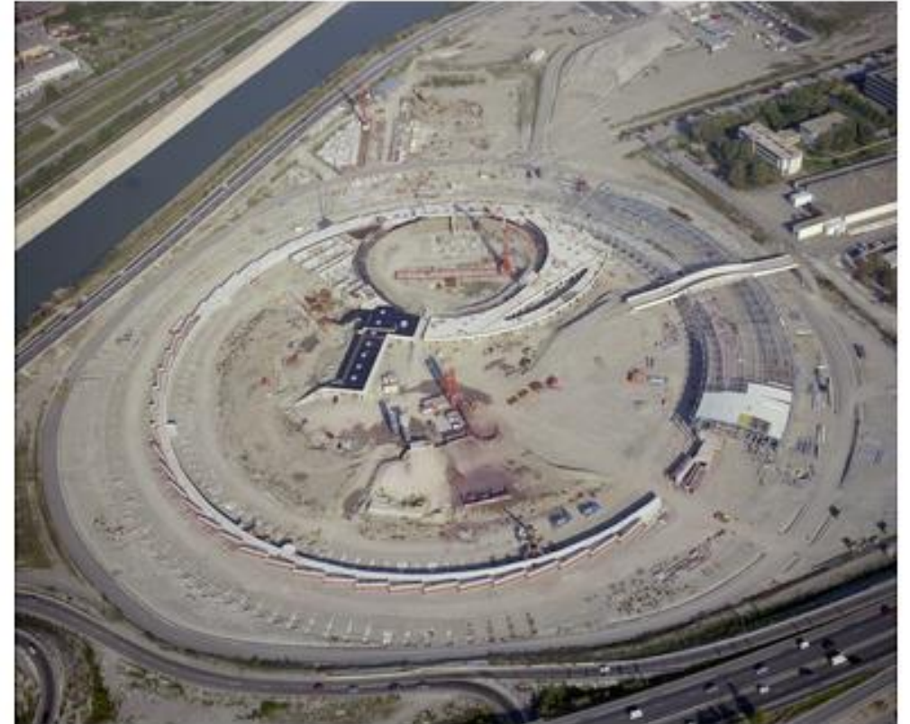
ESRF construction site, 1990
