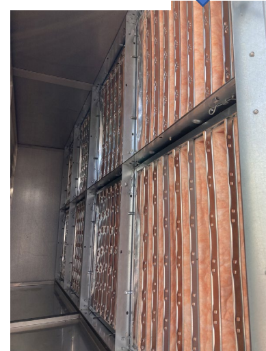
Air filters improvement
