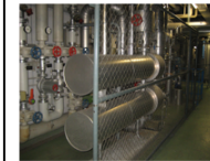
Existing heat exchanger with dT_m=22K
