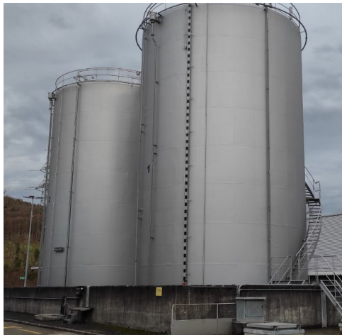
Oil storage tanks
