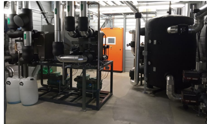
New chillers including buffer tank
