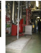
New heat exchanger with dT_m=5K
