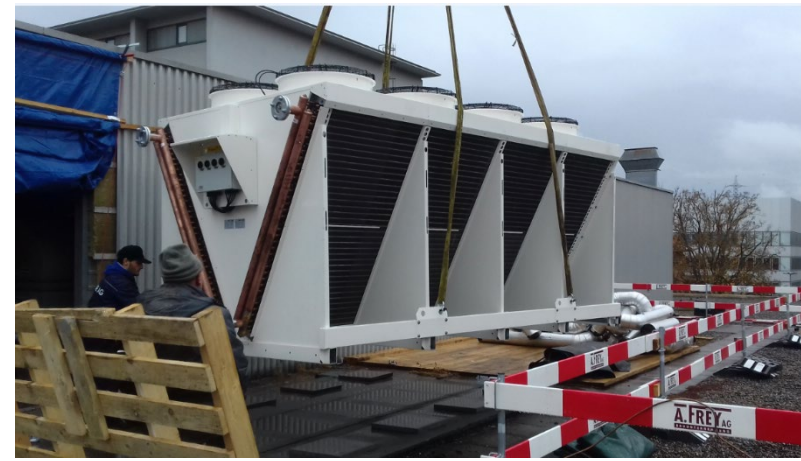
Assembly of dry cooling unit on the building roof
