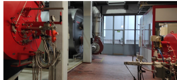
Heating boilers 30MW for backup 80MW district heating system)
