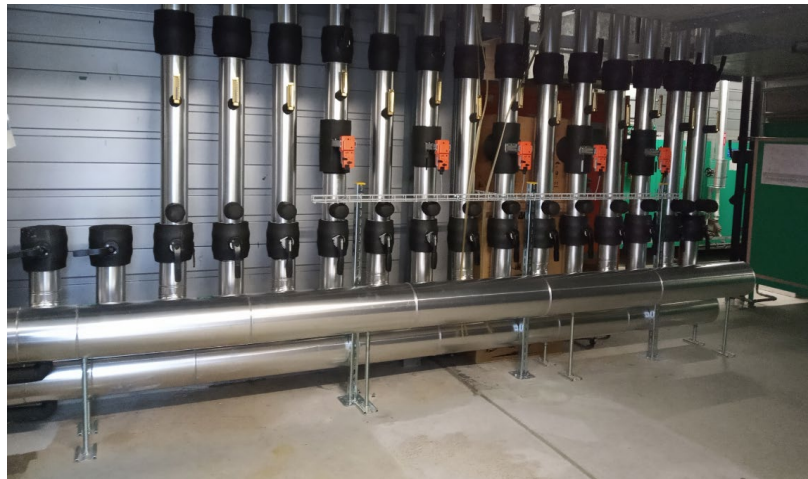
Cooling water distributor including emergency connection
